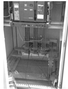
Fig. 2. Connection of current sensors in the field.
