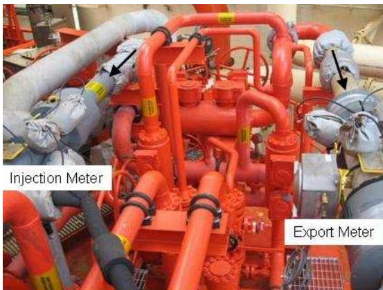
Fig. 2. Metering Station.
