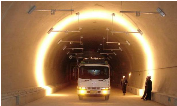
(b) Inspection system of the tunnel lining using CCD cameras (KMTL, Korea)
